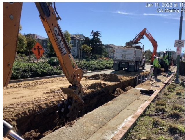
Installing pipeline on 2 nd Ave.
